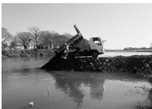
Fig. 9 Carry in contaminated soil in cleaning pond
