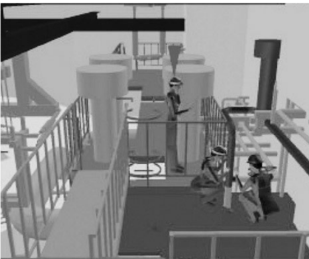
Fig. 5 Simulation of removal work of helium system piping in reactor building of Fugen
